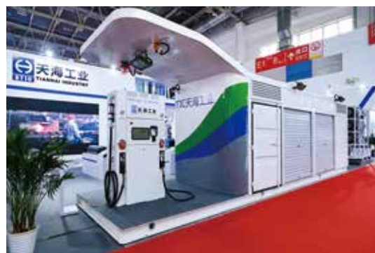
撬装式加氢站 Skid mounted hydrogen refueling station
